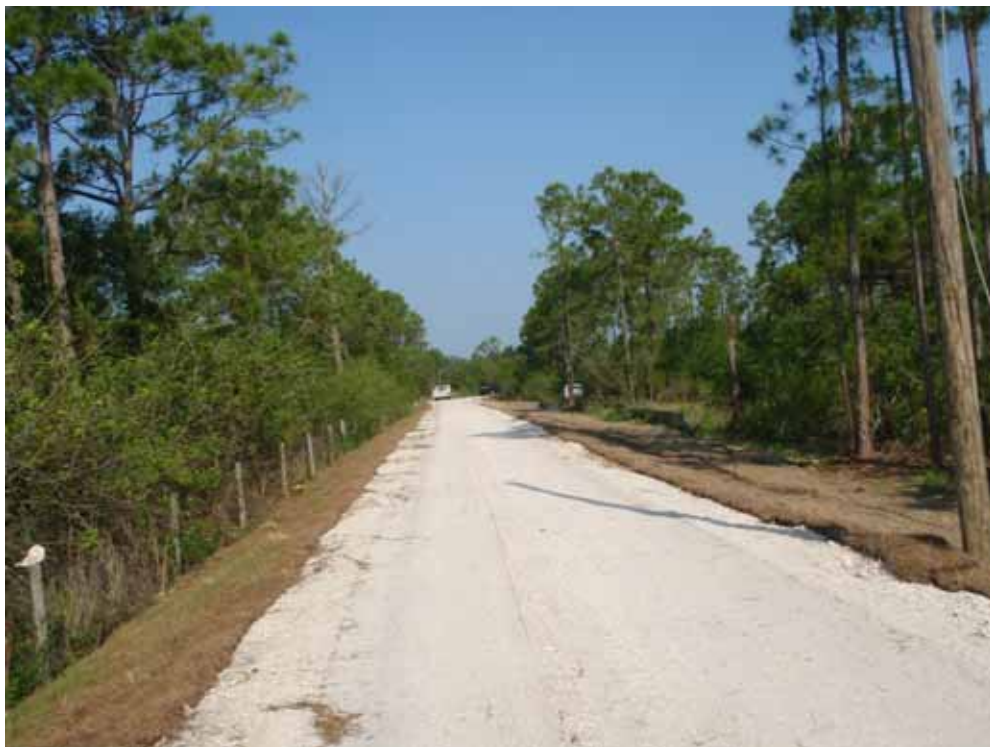
Photo #7. Now the berms are complete. They have put a shell rock on the tops and planted sod on the sides. Hopefully we will get rain soon so that the sod can get established, but for now the contractors are watering it with a truck.
