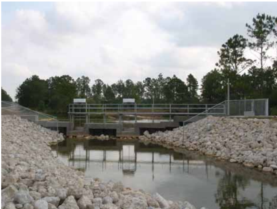
Photo #6. Although it is hard to see in this picture, sod has been planted around the weir. There is also a fence and protective boxes to prevent vandalism.
