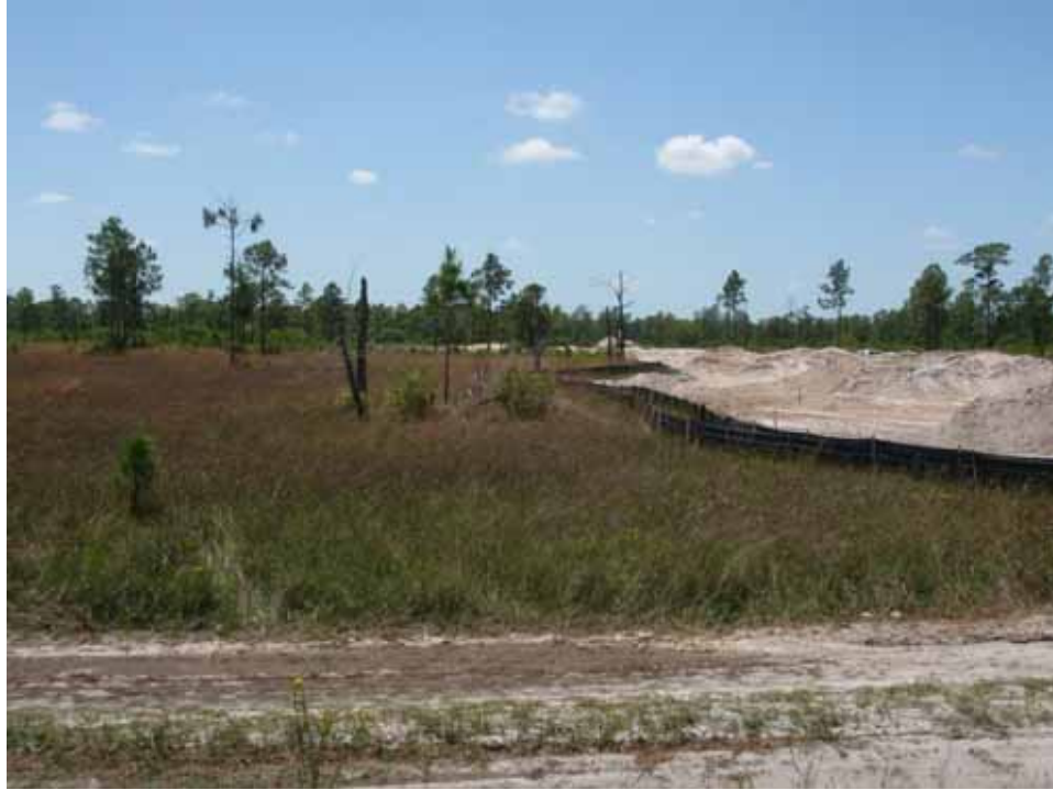
Photo #2, top soil returned to the flow way for the plantings. At this point it hasn't been spread out yet.
