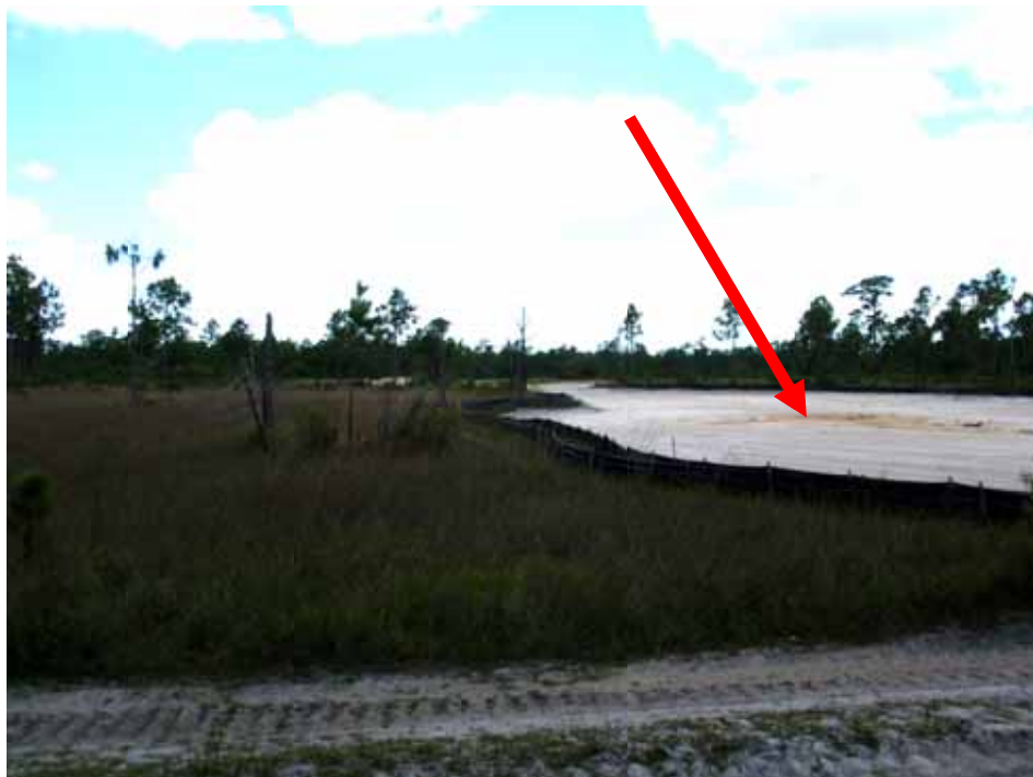
Photo #2, the top soil has been spread out to its final elevation. They have also installed several "fish traps" (red arrow). They are slightly lower areas that will hold water for longer periods, trapping fish for birds to eat.
